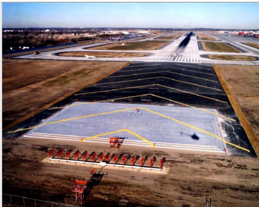
FIG 2-3-42 Engineered Materials Arresting System (EMAS)
